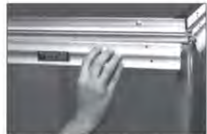
3. Attach front plate with machine screws provided. Your installation is complete.
