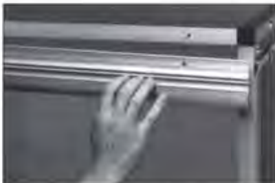
1. Mount the rear track. Hardware is provided for attachment to virtually any surface.
