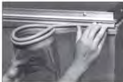
2. Unroll your new softwall panels and hook into place. Overlaps are automatic and strips are perfectly aligned every time.
